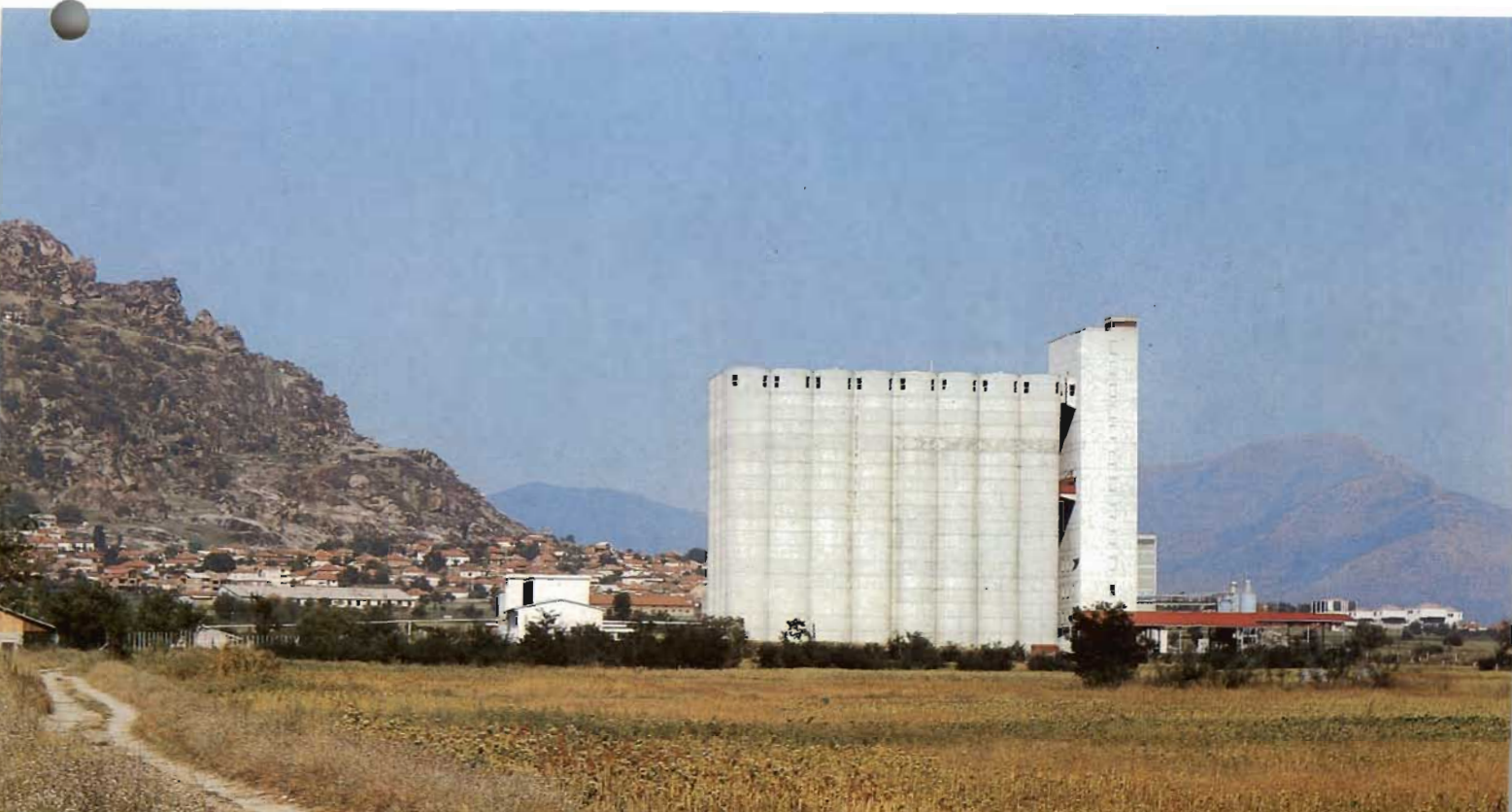
Concrete silo bins
