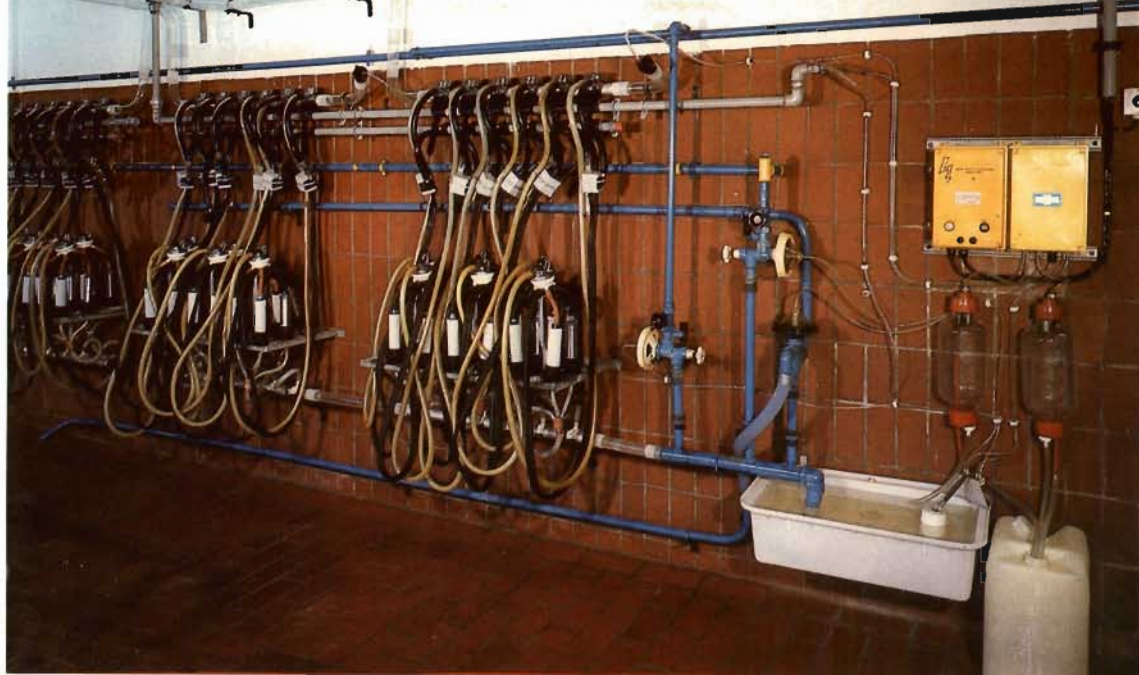
Milking cluster, disinfesting and cleaning installation
