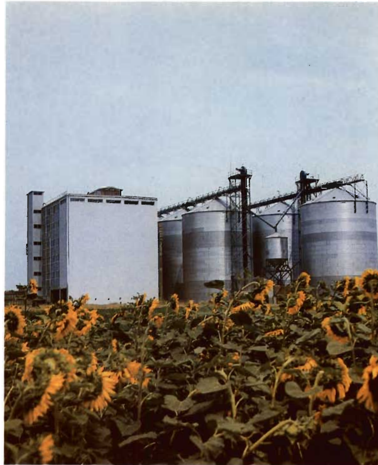
Metal silo bins
